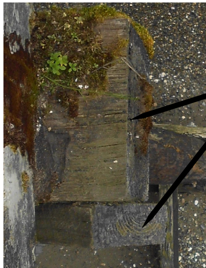
FIGURE 3B - PILECAP AND BRACE FLASHING
