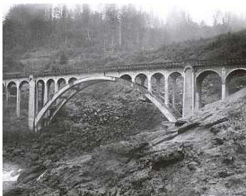
Ben Jones Bridge Photo: Reference 5
