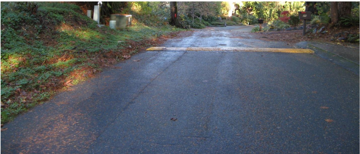
Figure 32. Landscaping has filled in the shoulder of the north side of roadway Raft Island Drive (Plot 4995000703).
