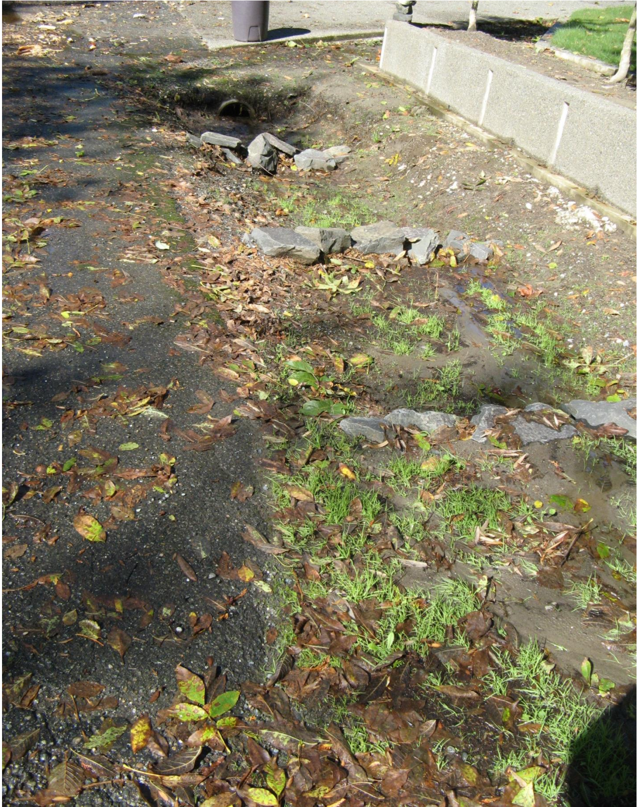
Figure 38. Shoulder on east side of Raft Island Drive filling through driveway drain with silt Raft Island Drive (Plot 4995100120).
