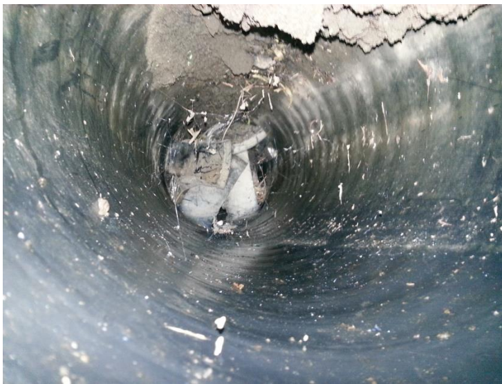
Figure 26. Crushed drain crossing Raft Island Drive at Adler (Plot 4995100630 to 499500820). Replacement needed.
