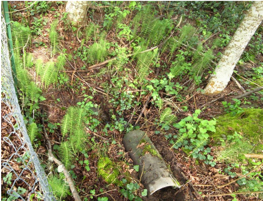
Figure 34. Drain needs catch basin and clearing on east side of Raft Island Drive. A possible community mail box (Plot 4995100490).
