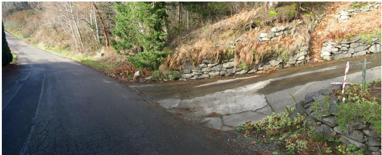
Figure 2. North side of road at 168 Raft Island Drive (plot 7097000131) water running down the driveway into the road. Note fatigue cracking on roadway.
