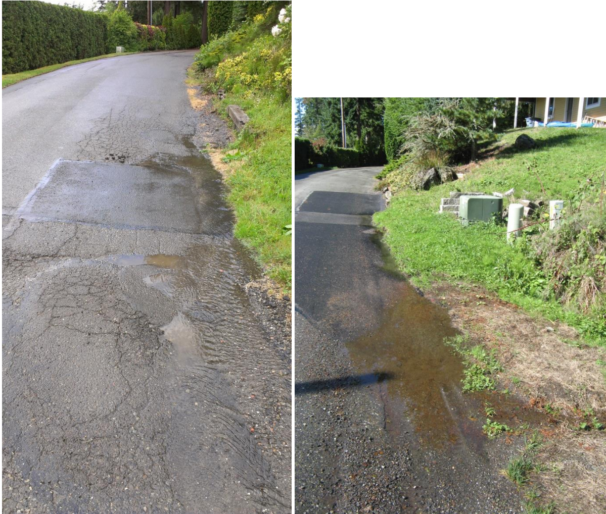
Figure 39. No shoulder drainage on East side of Raft Island Drive (Plot 4995100061).
