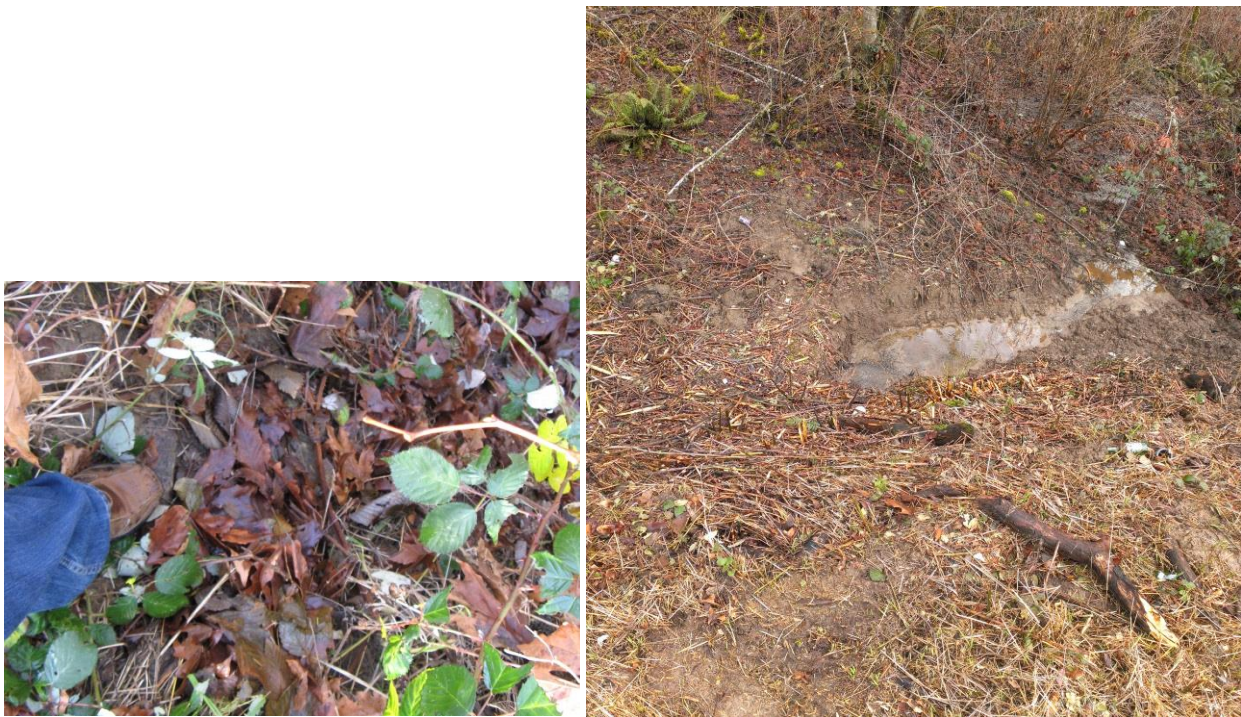
Figure 14. East side of road across from 184 Raft Island Drive (plot 7097000111) drain exit. Right image of post pipe end cleared.
