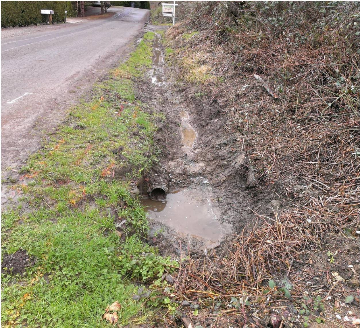
Figure 7. North side of road at 180 Raft Island Drive (plot 7097000191) Drain cleared by ditching 2015.01. Note French drain running parallel to the roadway (installed decades? before 2015). This was filled by current property owner 2015.10.
