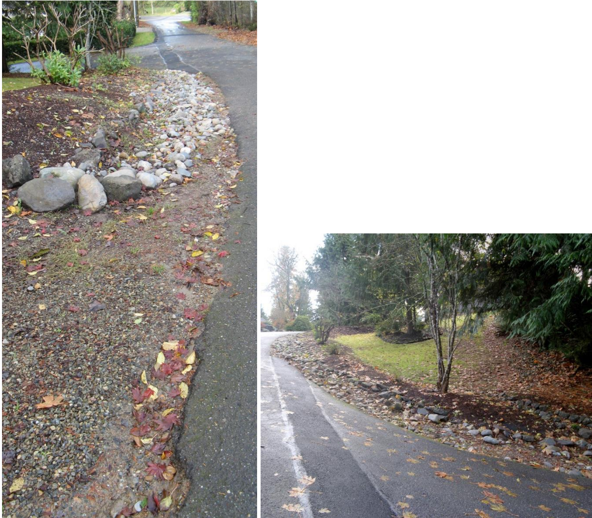
Figure 68. Gravel along West side of Fir Drive blocking good drainage and eroding the roadway. (Plot 4995100710)
