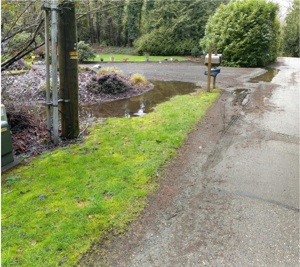
Figure 28. Poor drainage on south side of Raft Island Drive (Plot 4995100600).
