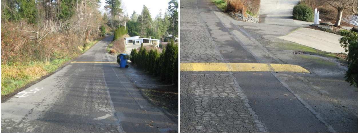
Figure 3. Raft Island Drive. Note fatigue cracking on roadway.
