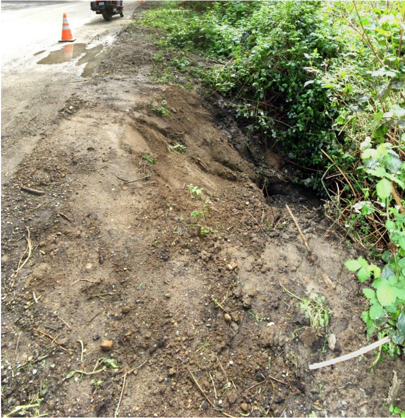
Figure 35. Drain exposed on west side of Raft Island Drive during water main replacement (Plot 4995001160).
