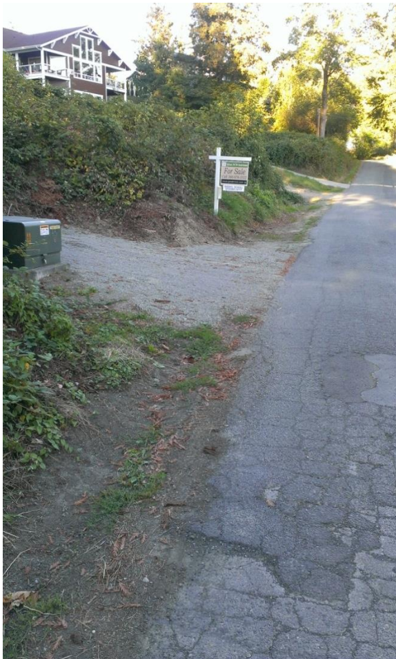
Figure 5. Raft Island Drive. Note fatigue cracking on roadway and lack of roadside drainage on north side. (plot 7097000052)
