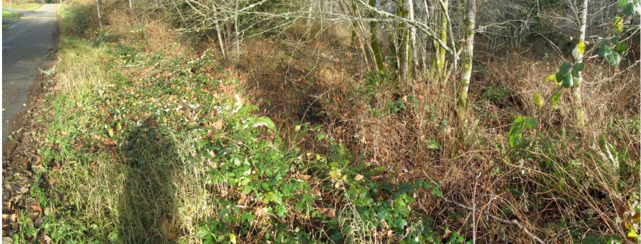
Figure 13. East side of road across from 184 Raft Island Drive (plot 7097000111) under road drainage exit.
