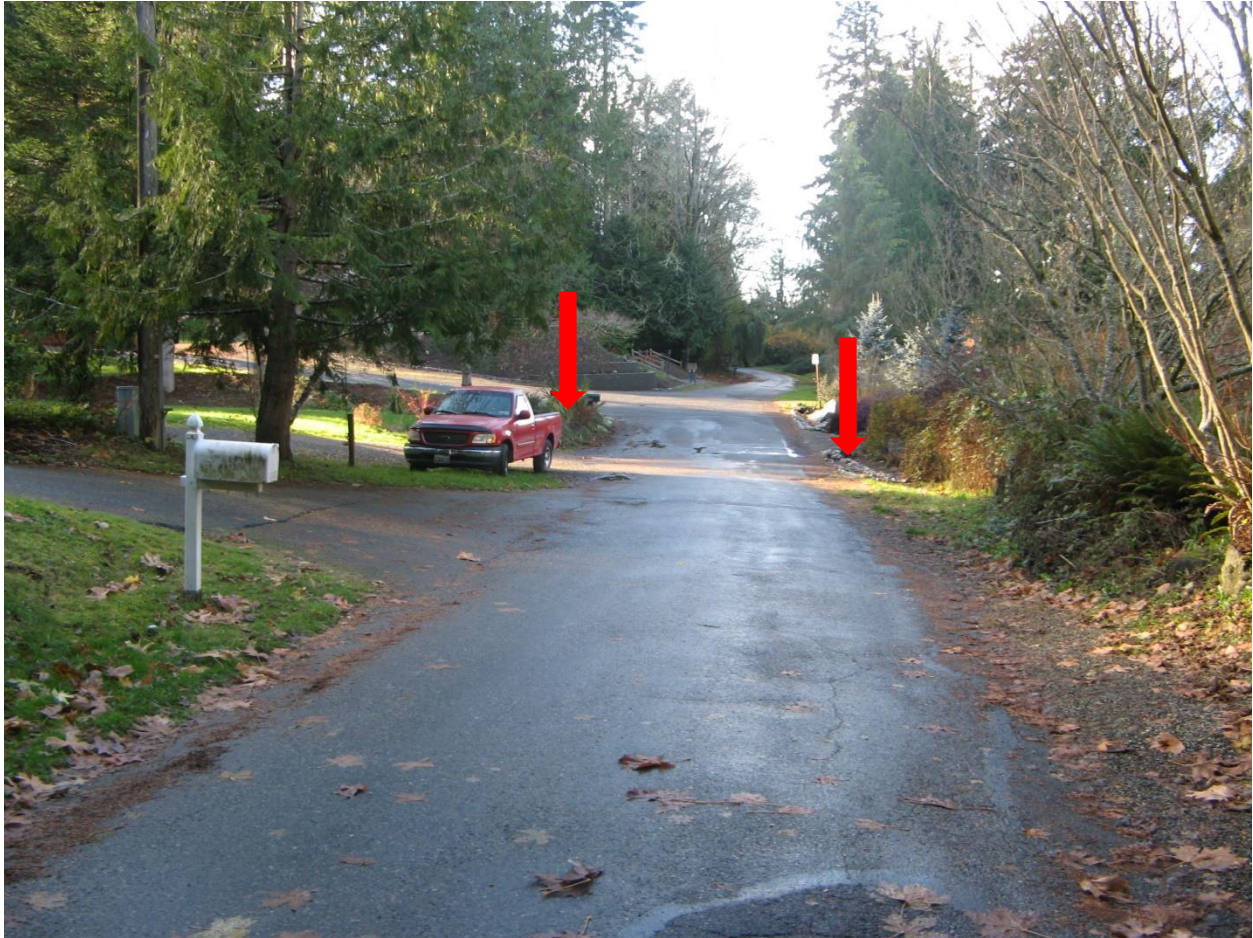
Figure 22. Raft Island Drive North East. Drain crossing Raft Island road at Fir Drive is not visible. Run off from Fir Drive draining over road.
