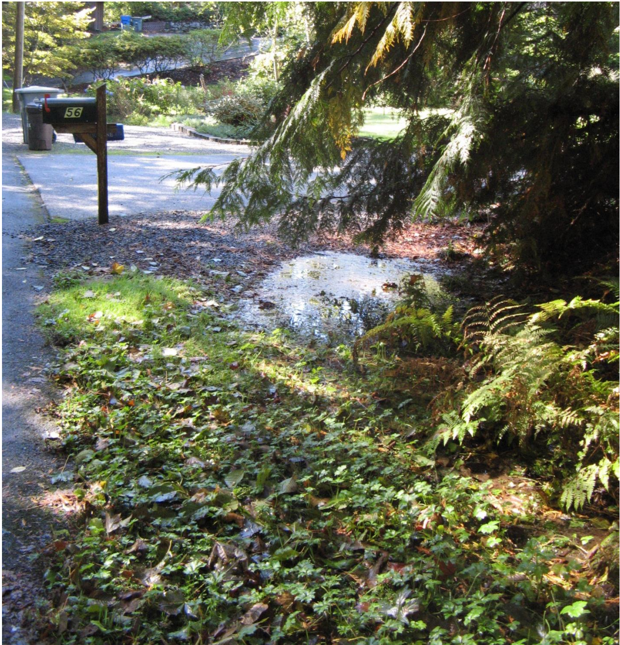
Figure 64. Poor drainage on North side of Park Avenue. (Plot 4995100452)
