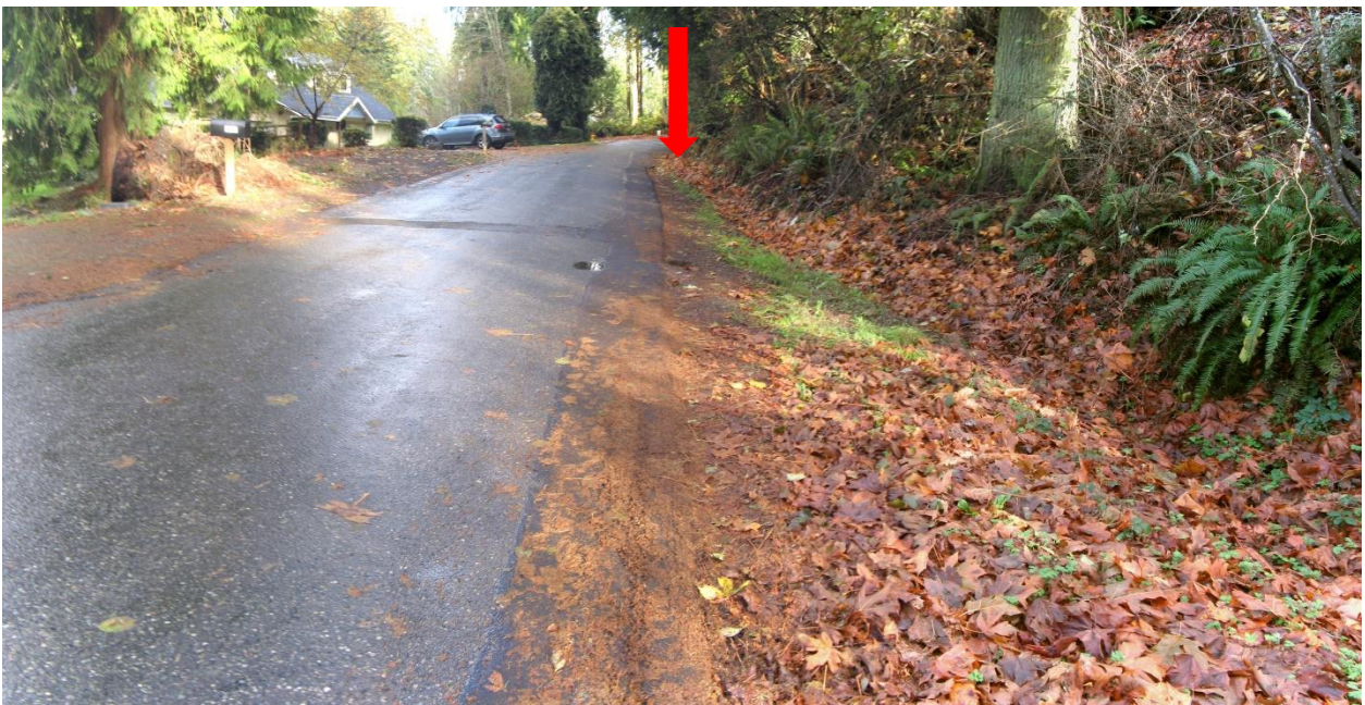
Figure 66. Roadside drainage adequate though drain is filled on South side of Park Avenue. (Plot 4995100700 and 4995100710)
