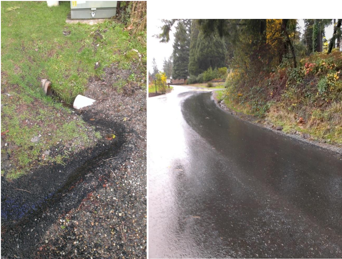
Figure 59. Drain at the East side of Madrona near Raft Island. Pipe end has been replaced and its full length cleared, 2015.01. Image on the right is before clearing showing runoff washing the shoulder's gravel. (Plot 7097000112)
