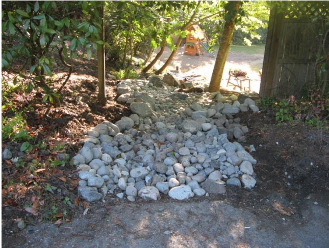
Figure 57. West side of the through road drain across Madrona Drive, entering lot 12 Rhododendron Drive following completion of the drainage repair project. (Plot 4995100202)
