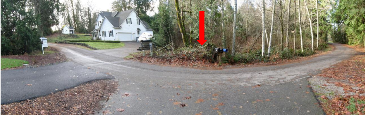
Figure 18. Raft Island Drive South East (drainage into plot 4995000220 from plot 7007000301). Drain pipe end concealed, filling with debris.
