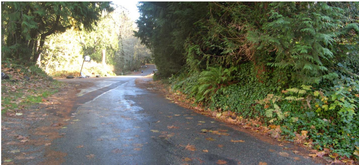
Figure 21. South side of Raft Island Drive across from Maple Lane, drainage at shoulder filled. (plot 4995001180).
