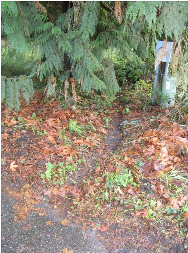
Figure 30. Drainage off the roadway south side of Raft Island Drive (Plot 4995100573).
