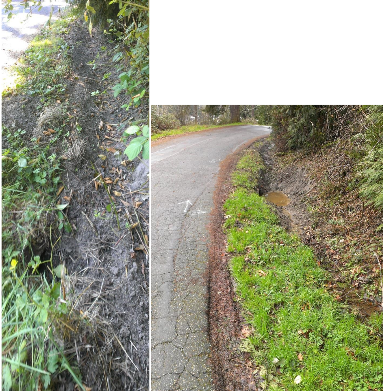
Figure 11. North side of road at 184 Raft Island Drive (plot 7097000111) ditching visible on right. Note fatigue cracking on roadway.
