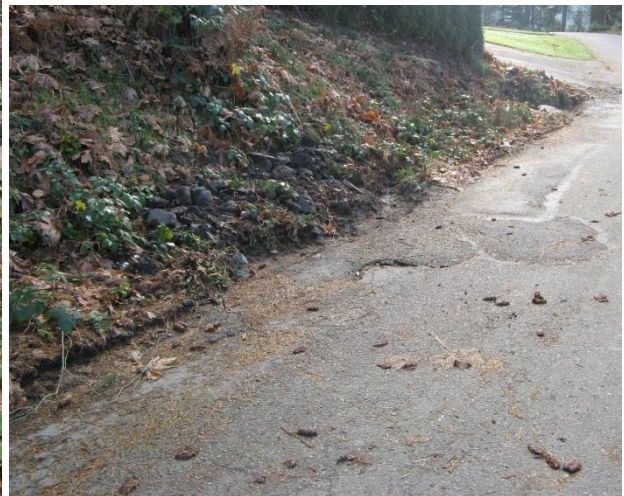
Figure 52. Madrona Drive east side of the road needs clearing for proper drainage. (Plot 4995100670)
