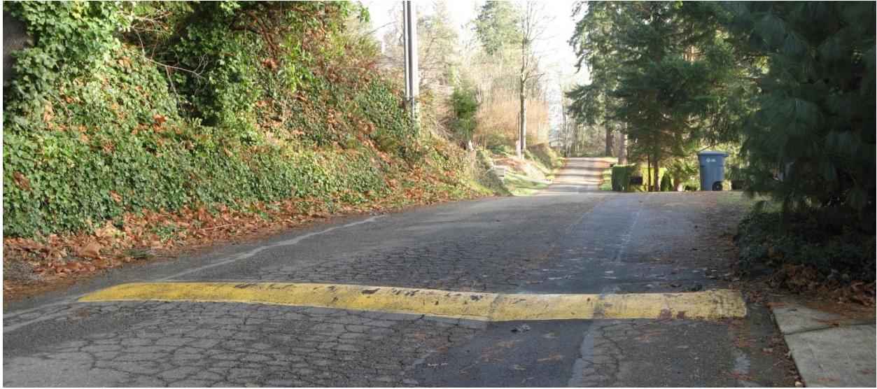
Figure 5. Raft Island Drive. Note fatigue cracking on roadway and lack of roadside drainage on north side. (plot 7097000052)
