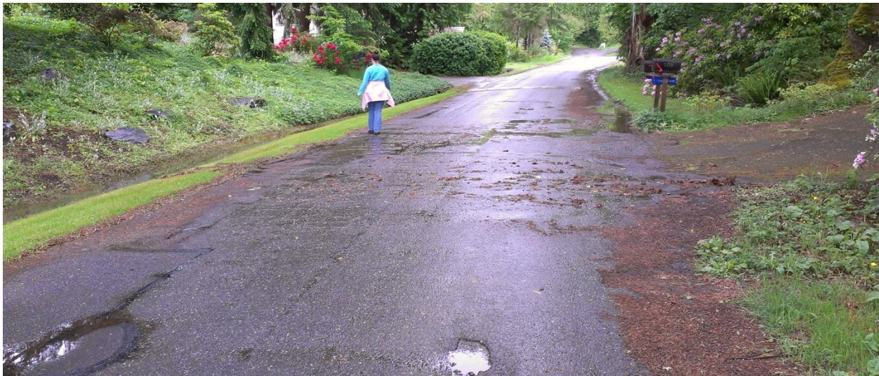
Figure 24. South side of Raft Island Drive drainage needs opening. (plots 499100630, 499500190, 4995001170). North side well maintained.
