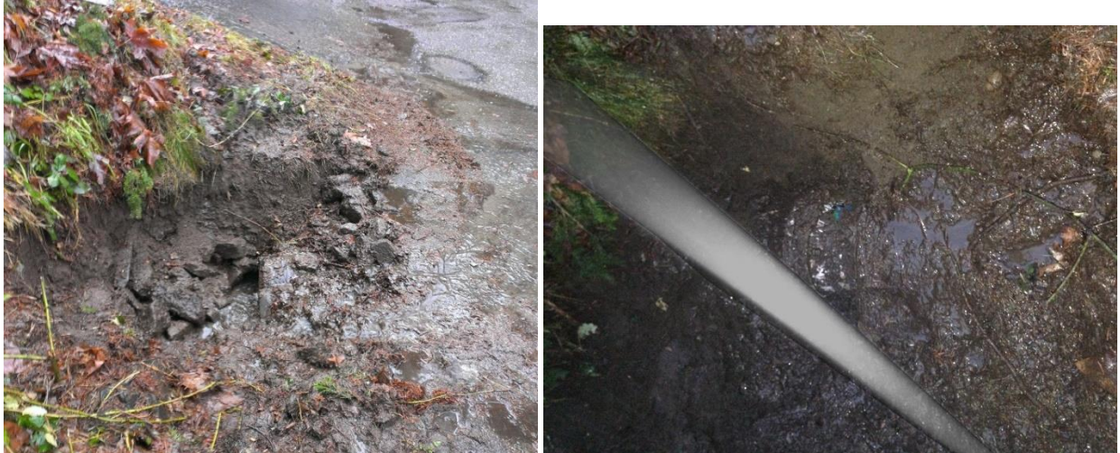
Figure 53. Madrona Drive east side of the road drain showing bucket after digging the end up. (Plot 4995100670)
