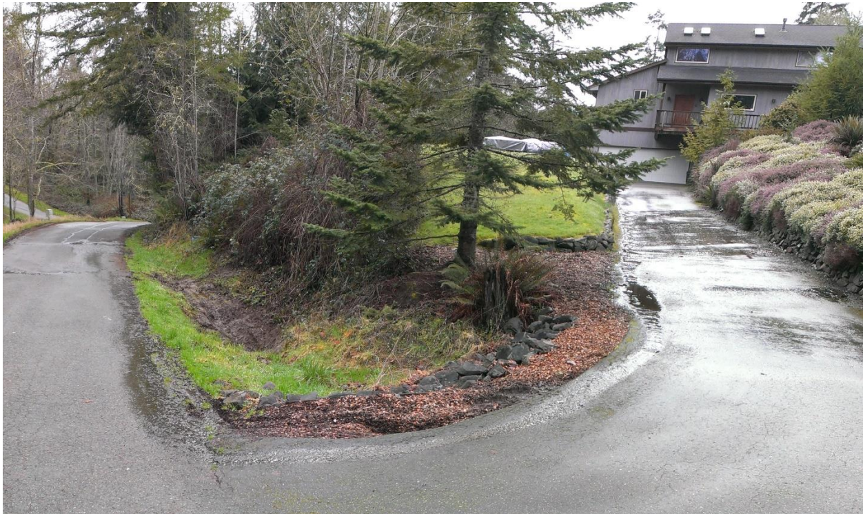
Figure 12. West side of road at 184 Raft Island Drive (plot 7097000111) under road drainage. Image on right shows post pipe end clearing. Runoff from drive way directed into the roadway. Note fatigue cracking on roadway. Water should be directed into the roadside ditch.
