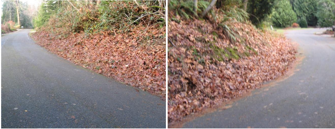
Figure 62. Roadside drainage filled on north-east side of Rhododendron Drive. (Plot 4995100240 and 4995100230)
