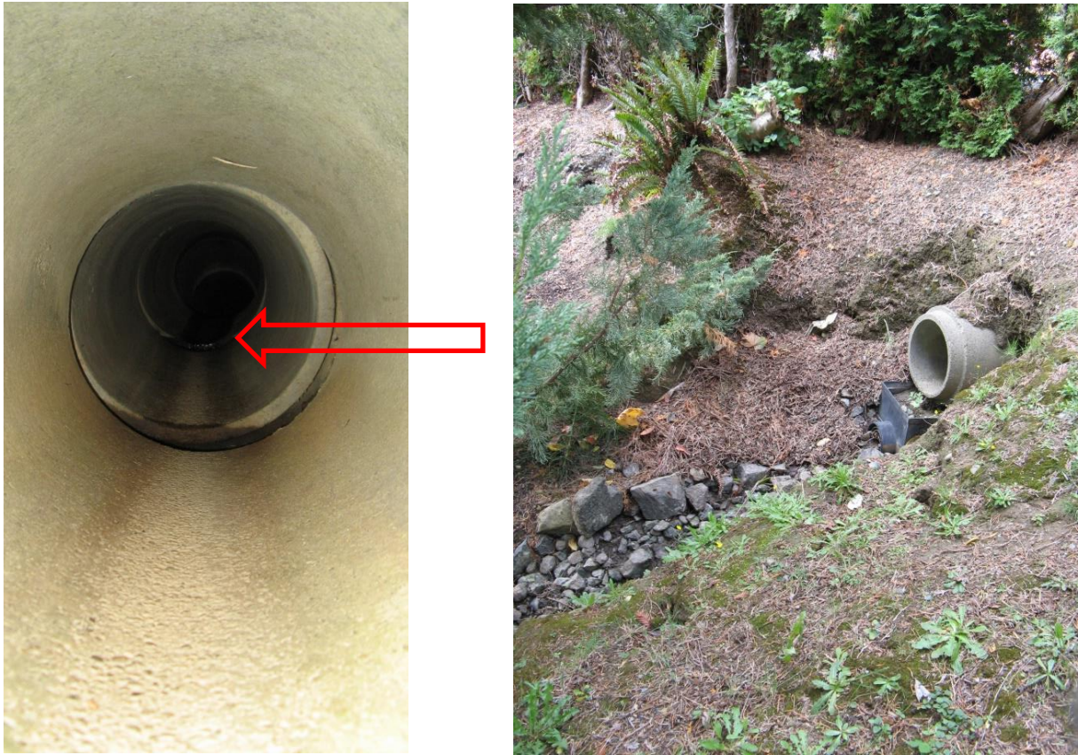
Figure 10. Drainage pipe separating and need replacing (plot 4995000360).
