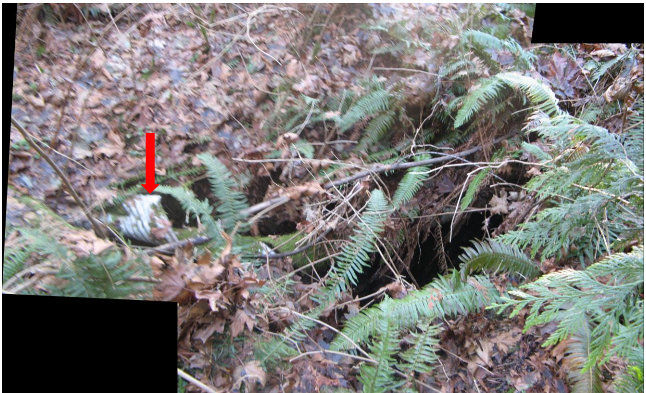
Figure 17. Raft Island Drive South East (drainage into plot 4995000220). Drain pipe broken, washing embankment away.
