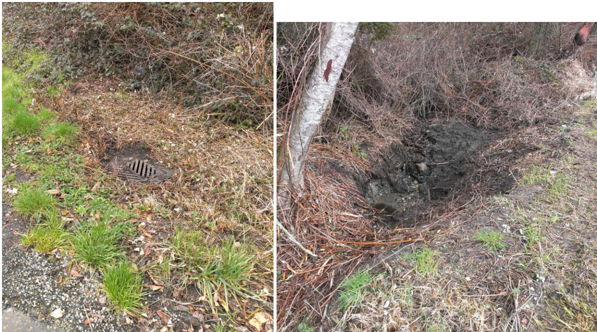
Figure 4. Raft Island Drive. Drainage near the areas shown above.
