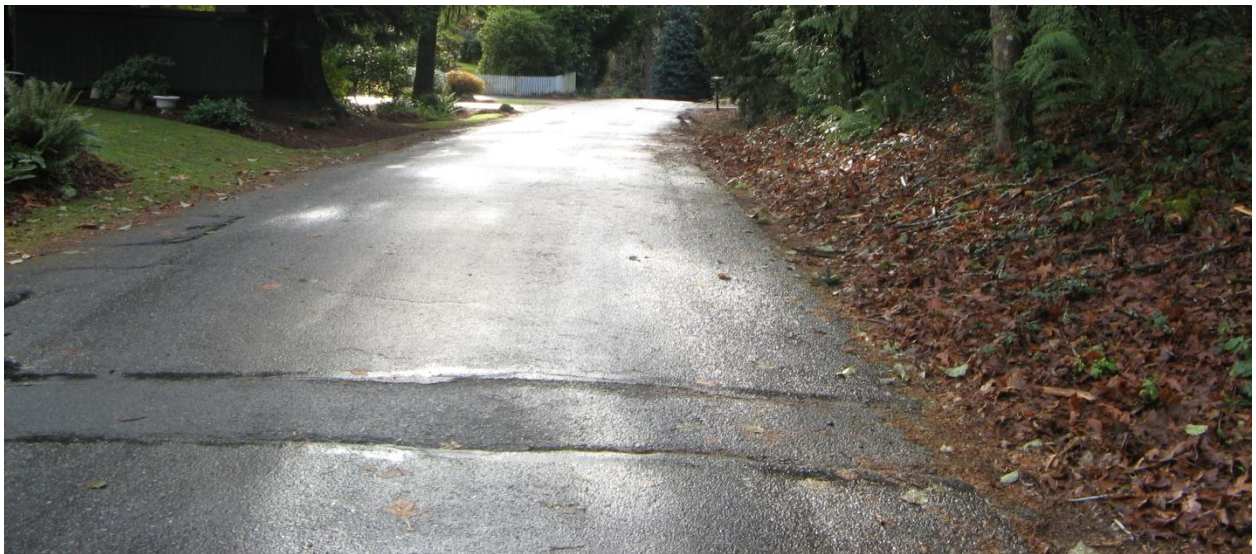
Figure 50. Poor drainage along West side of Madrona Drive. (Plot 495100690)
