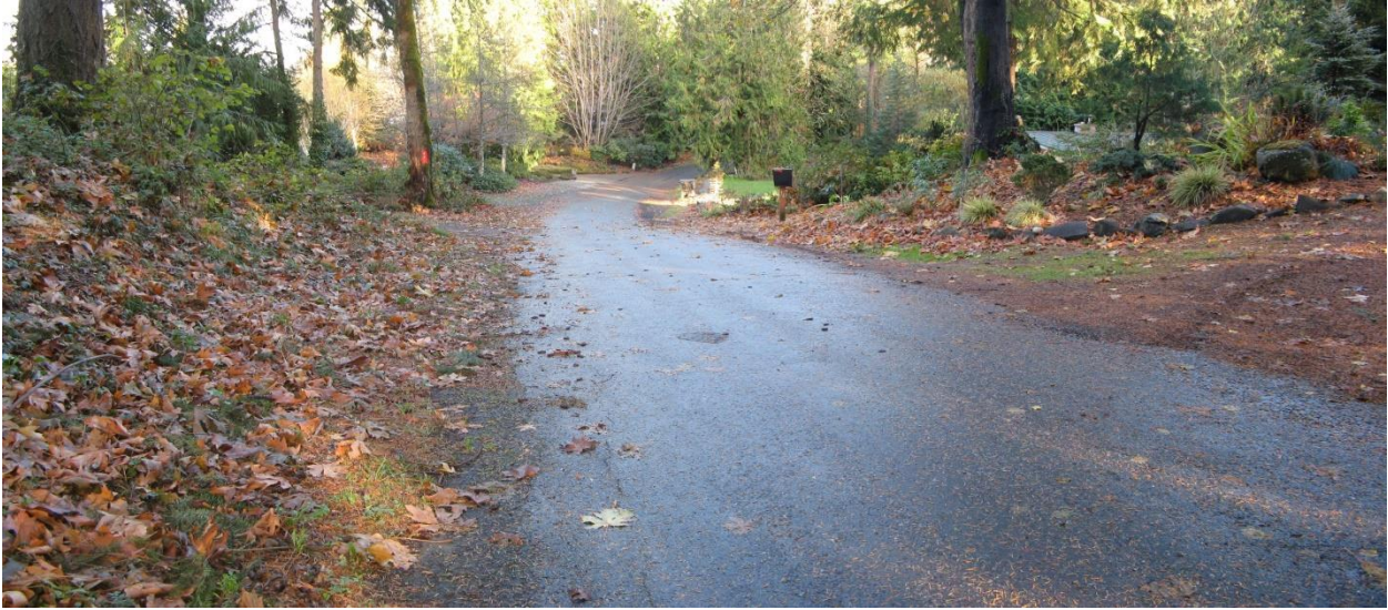
Figure 31. Landscaping has filled in the shoulder of the north side of roadway Raft Island Drive (Plot 4995000703).
