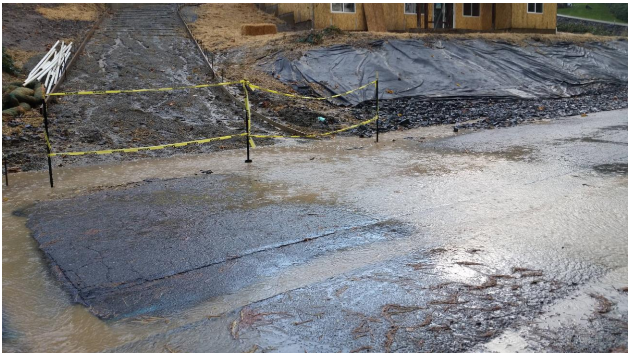
Figure 9. Lot 180 culvert covered with gravel. Owner to remove and clear drainage pipe 2015.11.01.
