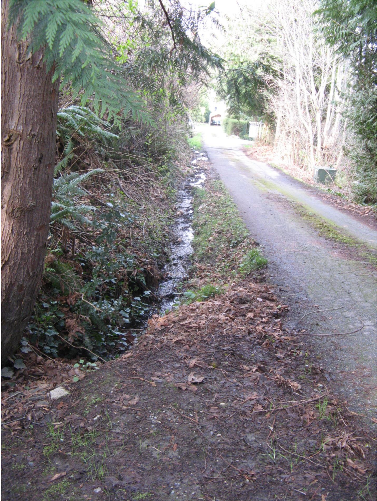
Figure 46. Poor drainage on South side of Maple Lane. (Plot 4995000841)
