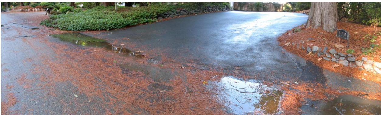
Figure 27. Drain plugged at driveway Raft Island Drive (Plot 4995000740).
