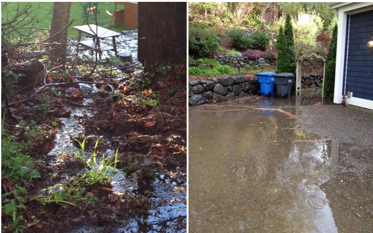
Figure 54. Flood through lot 12 and into lot 14 Rhododendron Drive. (Plot 4995100202 and 4995100181)
