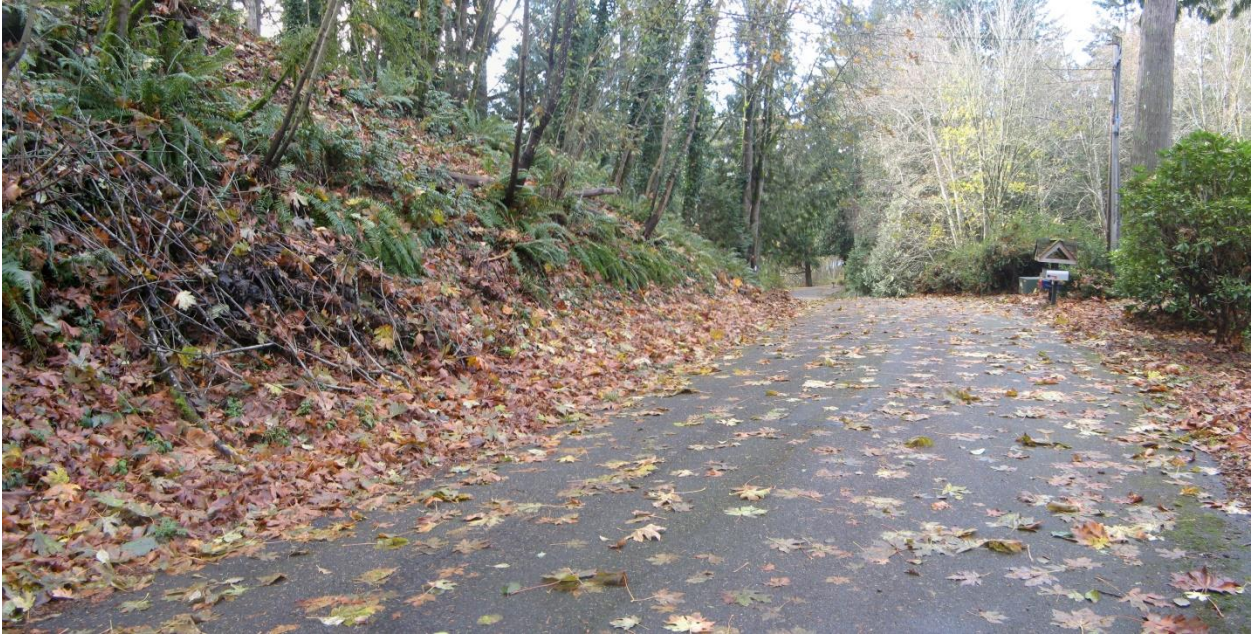
Figure 65. Roadside drainage filled on South side of Park Avenue. (Plot 4995100290)
