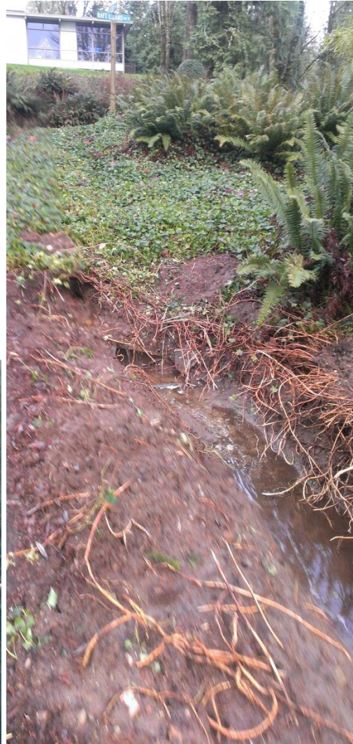
Figure 26. Crushed drain crossing Raft Island Drive at Adler (Plot 4995100630 to 499500820). Replacement needed.
