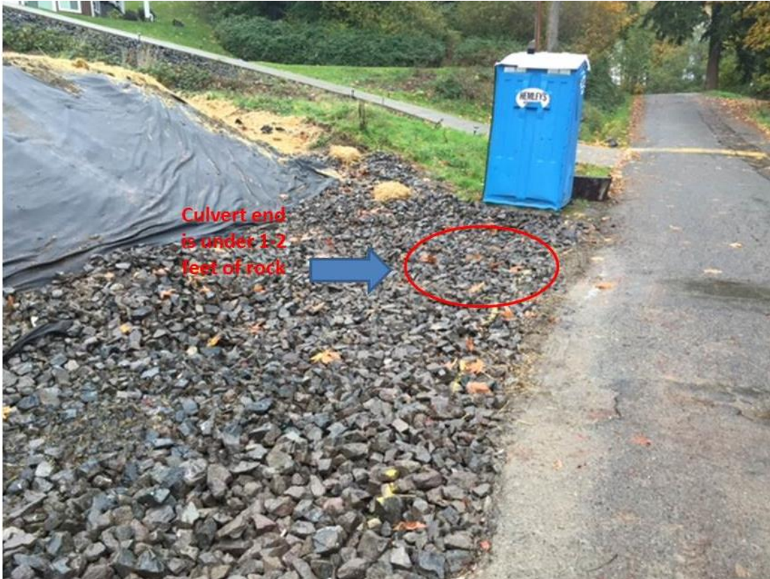
Figure 8. Lot 180 culvert covered with gravel. Owner to remove and clear drainage pipe. 2015.11
