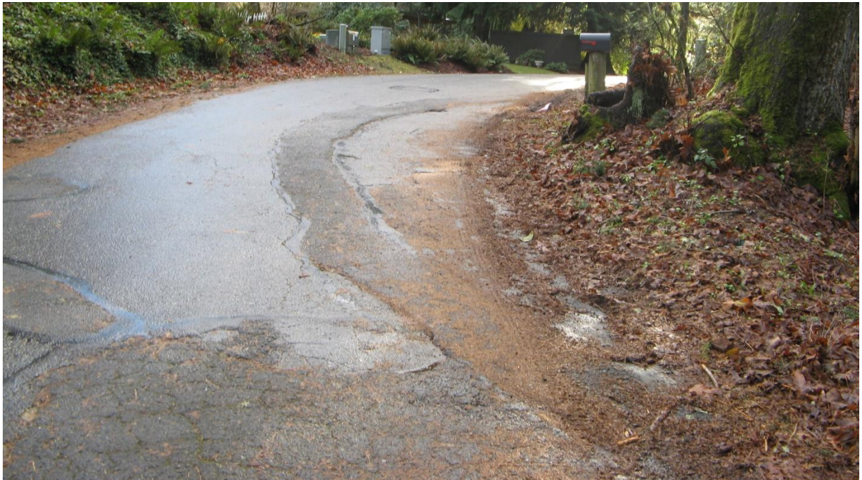
Figure 49. Poor drainage along Madrona Drive. (Plot 4995100310 and 495100700)
