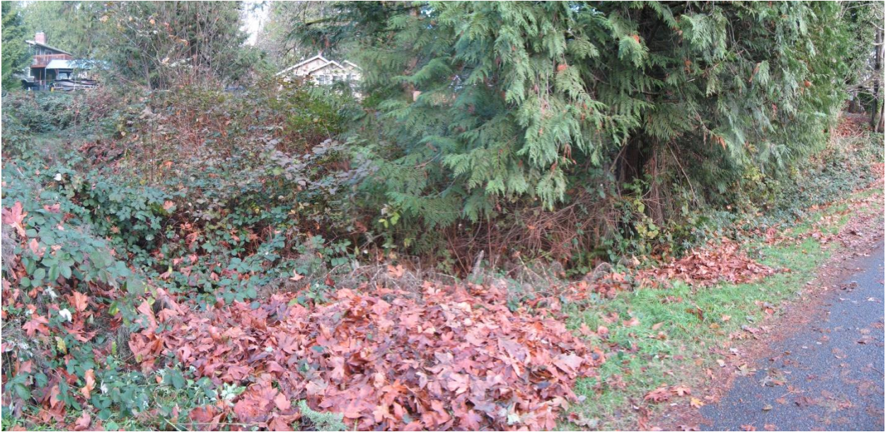
Figure 69. Drain on North side of Fir Drive needs clearing and catch basin. (Plot 7097000221)
