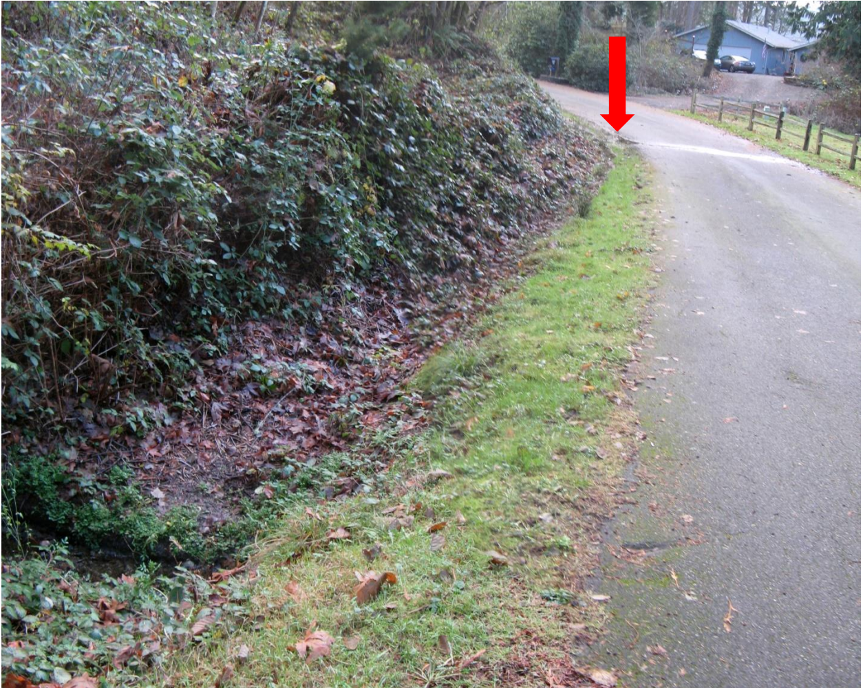
Figure 61. Drainage needs more slope on East side of Rhododendron Drive, near the intersection of Park Avenue. (Plot 4995100261)
