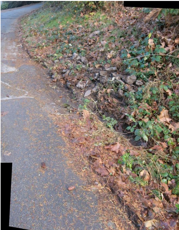
Figure 52. Madrona Drive east side of the road needs clearing for proper drainage. (Plot 4995100670)
