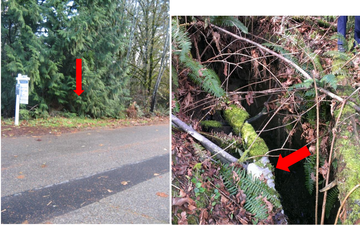
Figure 16. Raft Island Drive South East (drainage into plot 4995000220). Drain pipe broken, washing embankment away.
