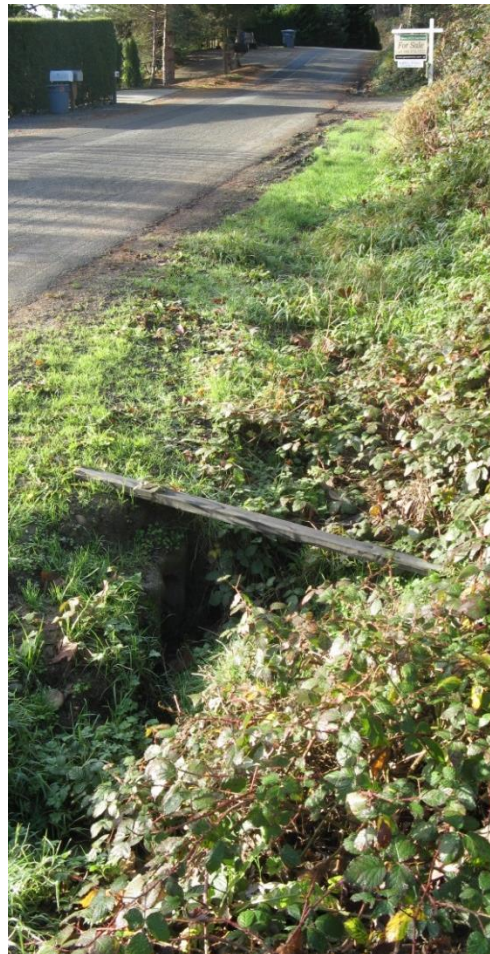
Figure 5. Raft Island Drive. Note fatigue cracking on roadway and lack of roadside drainage on north side. (plot 7097000052)
