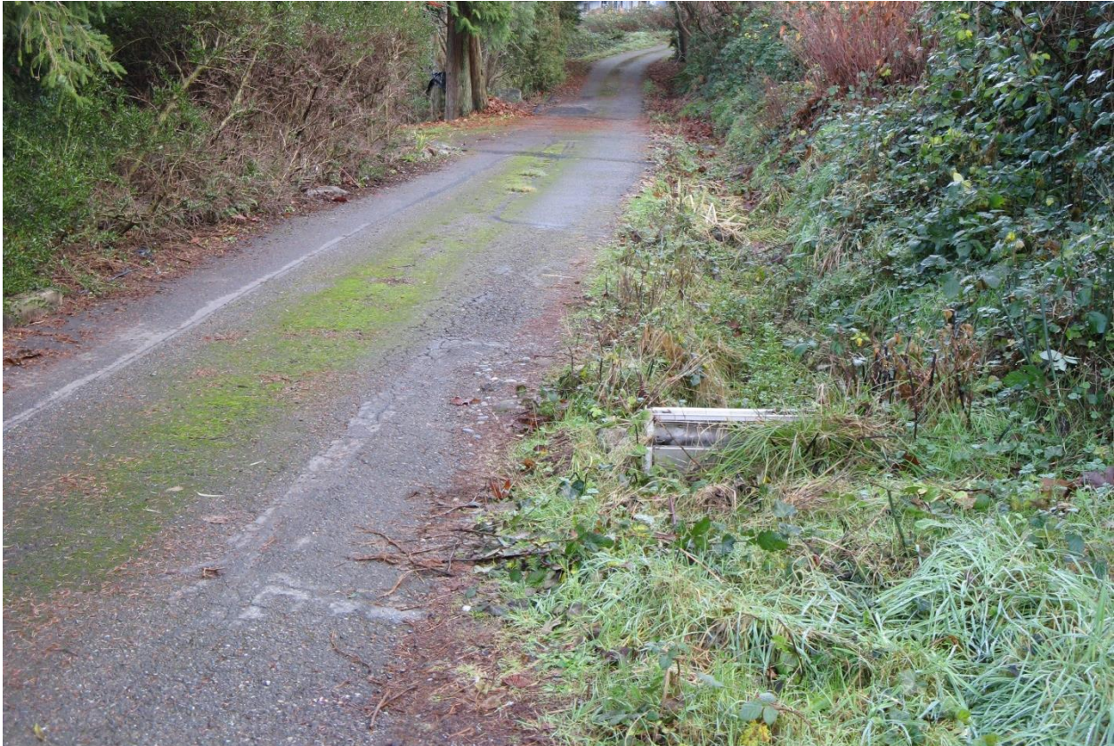
Figure 42. Alder Drive on 2014.12.13. Some sloughing of the hill, mostly overgrowth of vegetation.
