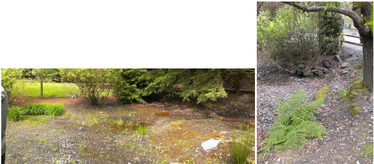
Figure 56. Eastern drainage pond and west end of the under driveway drain of lot 14 Rhododendron Drive. (Plot 4995100181)
