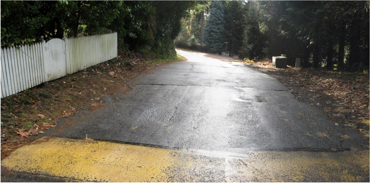
Figure 51. Poor drainage along Madrona Lane. (Plots 4995100680 and 4995100220)
