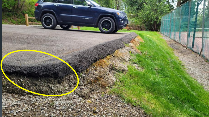
1. Parking starting to slough on the edges
