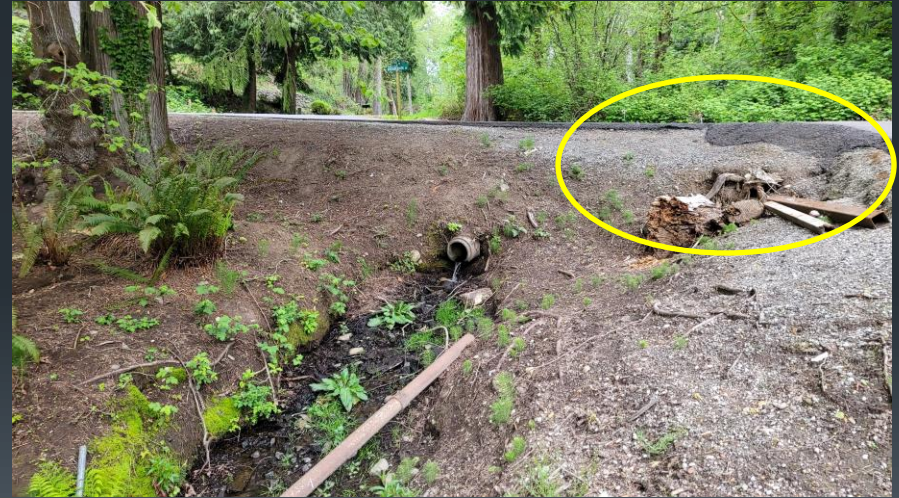
2. Roadway edge is starting show signs of sloughing into the ditch
