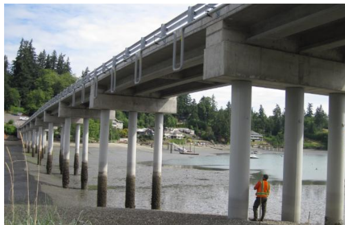
Photo 1 – Engineer completing Bridge Inspection.
