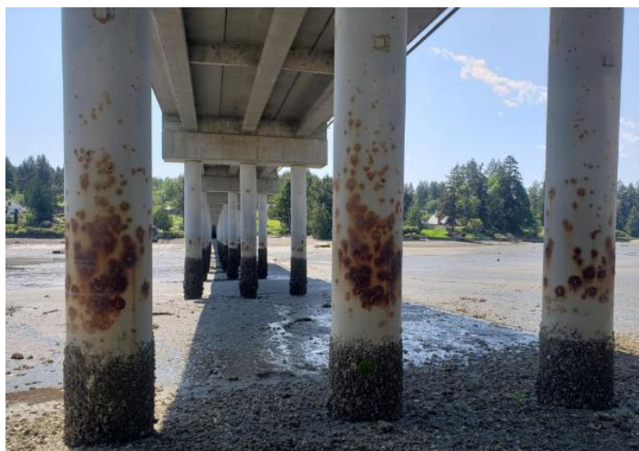
Photo 2. Piling at north end of bridge.
