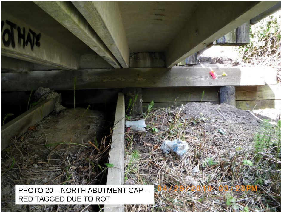
PHOTO 19 – NORTH ABUTMENT CAP – RED TAGGED DUE TO ROT
