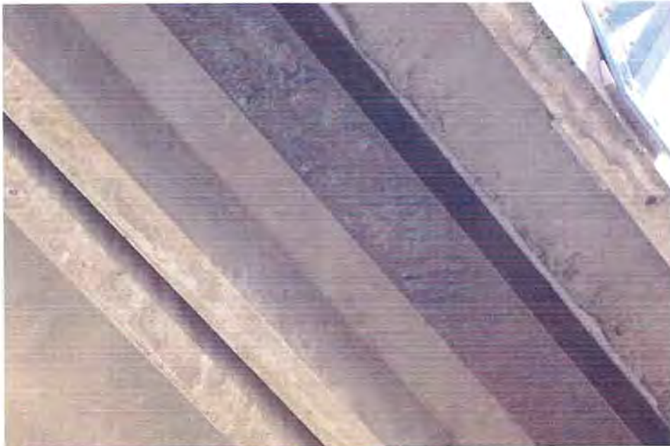
PHOTO 15 – GIRDER 42A RUST INHIBITOR PAINT ON STRENGTHENING BEAM
