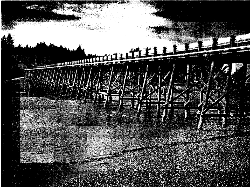
East Side View of Bridge
